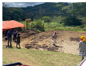
The leveled church ground
